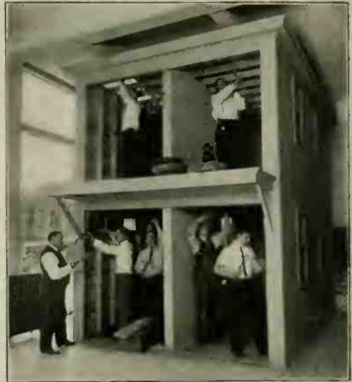
Training Future Electricians in a Miniature House in Which They Drill Beams, Put Up Cleats, Run Conduit, and Perform All the Other Tricks of the Trade Which the Practical Man Must Learn.
